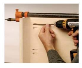
**7** Clamp sides to the bottom and drive the pocket screws. Then, lay the top upside down, position the cabinet on it and secure with screws.
