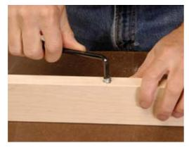
**4** Bore pilot holes for the 1/4-in. threaded inserts in the outer edge of each leg. Use a 6mm Allen wrench to drive the inserts into the holes until they're flush.
